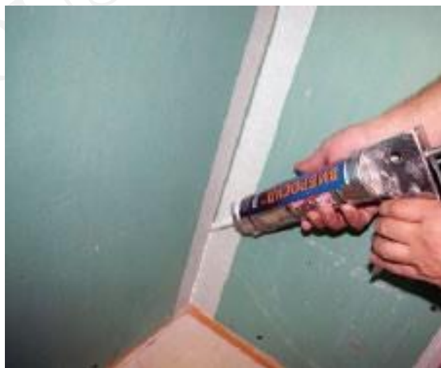
Figure 23. Filling the joints with Vibroseal sealant.
