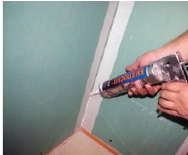
Figure 21. Filling joints with sealant.
