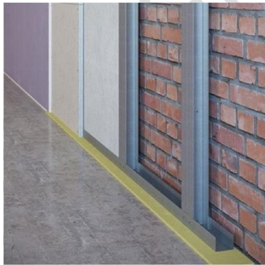
Figure 1. Image of 50/75/100 mm independent frame soundproofing cladding.
